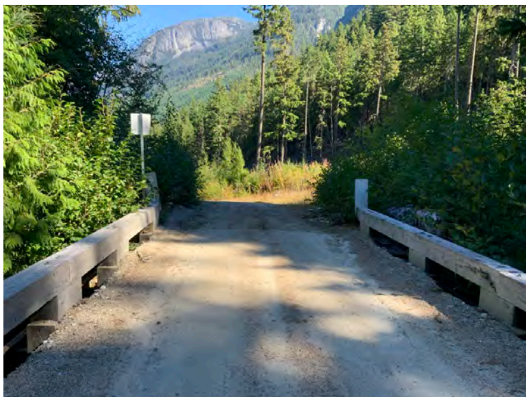
Approach from Right Bank when facing downstream
