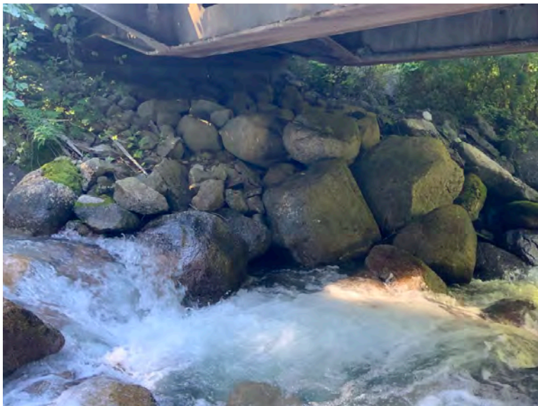
Left Bank Abutment when facing downstream
