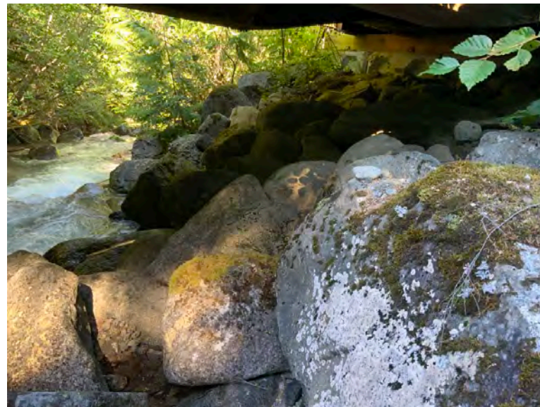
Right Bank Abutment when facing downstream
